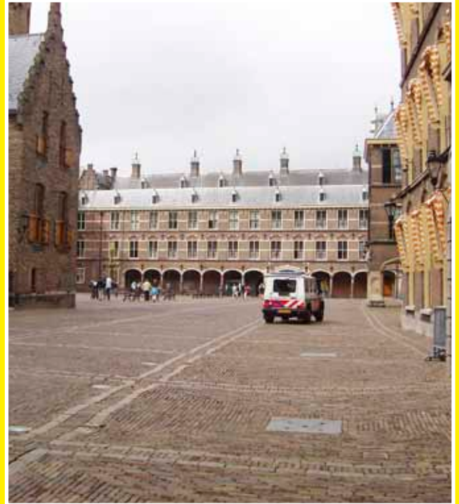
Offices of the Council of State
